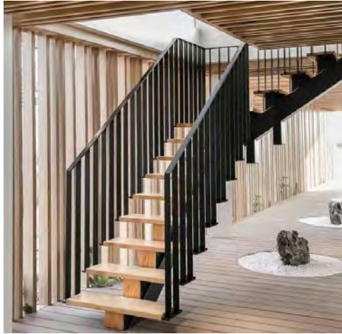
L Shape of Staircase
